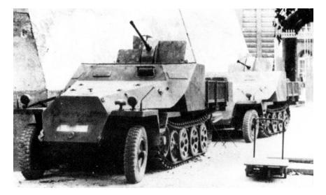
The Sd.Kfz.11 (though some sources name this vehicle Sd.Kfz. 30, Sd.Kfz.261, or Sd.Kfz.251/17 Neu) was one of many conversions, utilizing the Sd.Kfz.251 halftrack chassis and Flak.30/38 Anti-Aircraft Gun.
